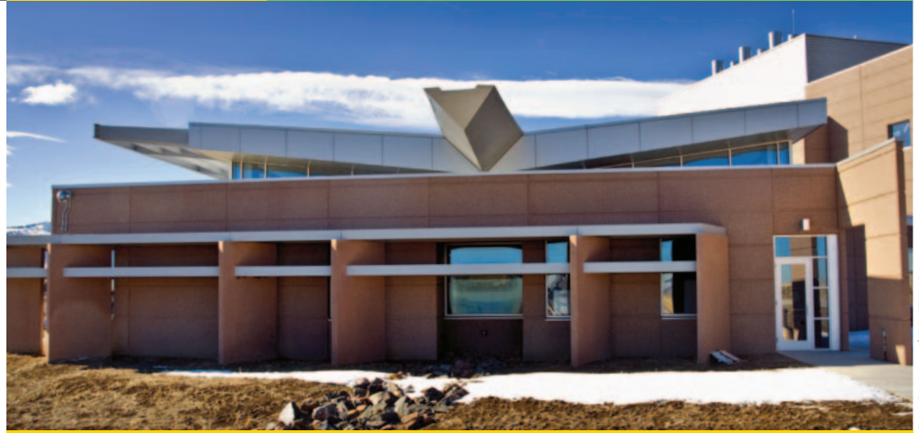
The Science & Technology Facility at the National Renewable Energy Laboratory in Golden, Colorado, incorporates a number of advanced energy efficiency and green building concepts. For example, the architecture makes good use of natural light wherever possible, and an automated system dims unnecessary artificial lighting to reduce electricity use.
