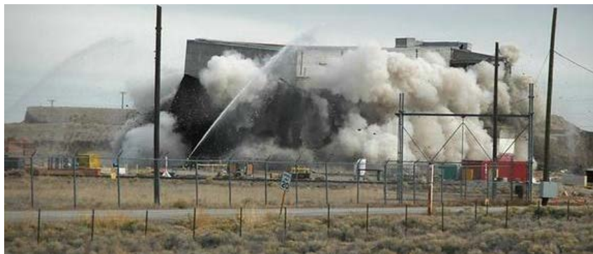
Idaho facility demolition
