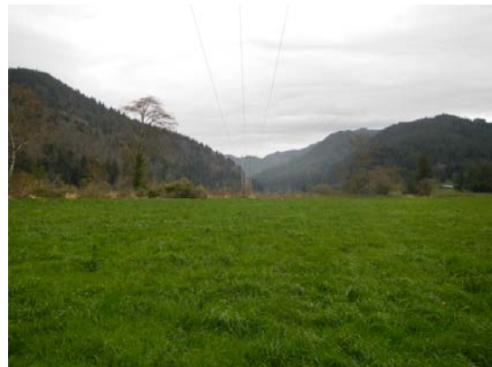
Structure 55/5 (Forest Grove-Tillamook No. 1) in background. ROW is pasturelands used for cattle grazing. Coast Range in background. Forest hillsides mostly red alder and western hemlock.
