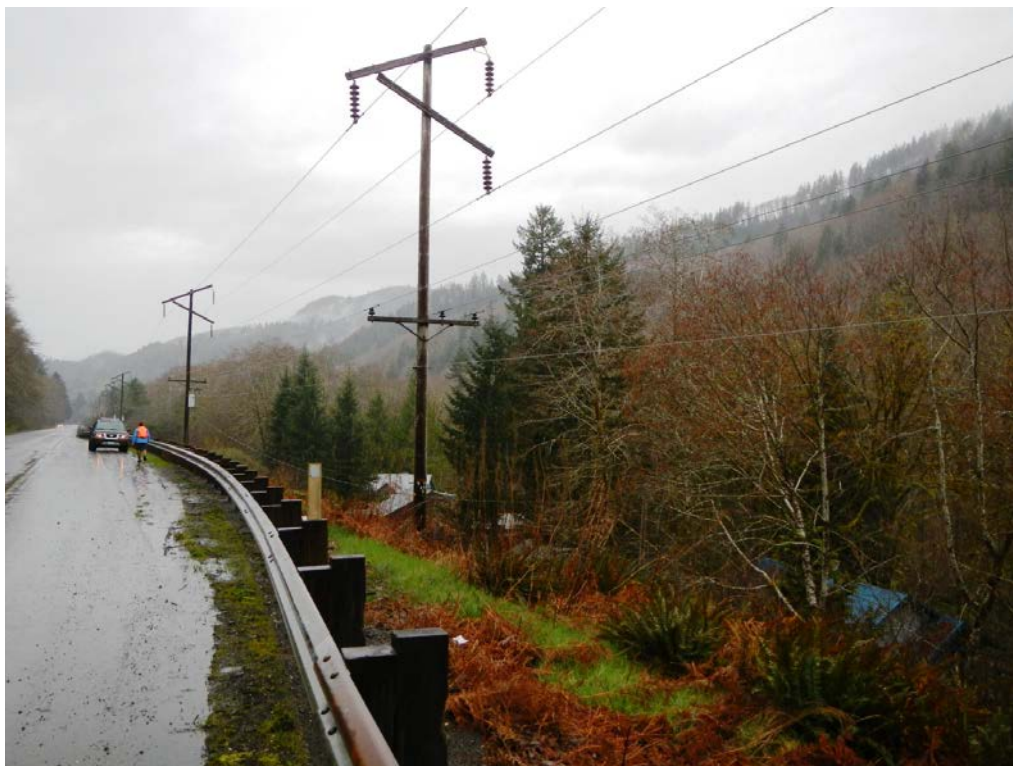
Figure 2-1. Existing Forest Grove-Tillamook No. 1 Transmission Line
