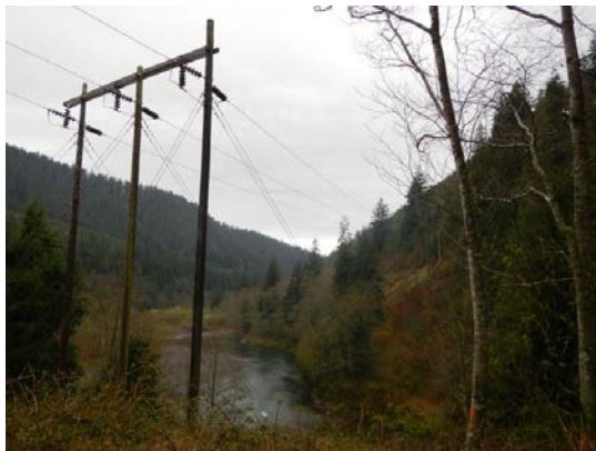
At structure 54/2 (Forest Grove-Tillamook No. 1). Transmission line crosses over the Wilson River. Blackberry thicket under lines. Danger trees on right, small alder trees marked with orange paint.
