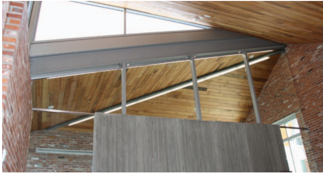
Daylighting built into the roof helps offset electrical lighting needs.
