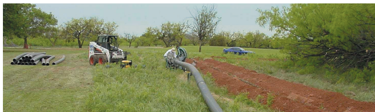
Work done under an energy savings performance contract enables Dyess Air Force Base to use Abilene’s effluent water for irrigation, saving 160 million gallons of potable water and $300,000 a year. Fusion-welded polyethylene piping connects Abilene’s effluent supply line to a holding reservoir on the base.
