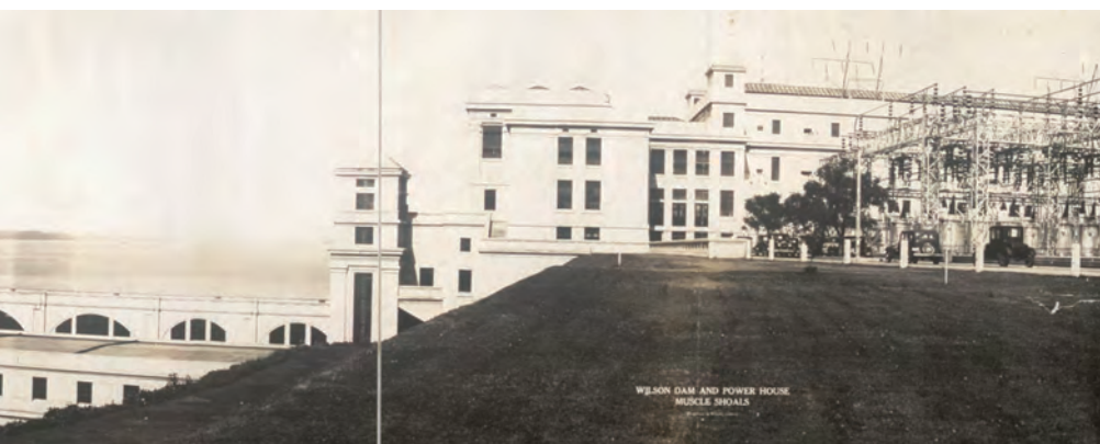
hydropower project in the southeastern United States (Library of Congress photo).
