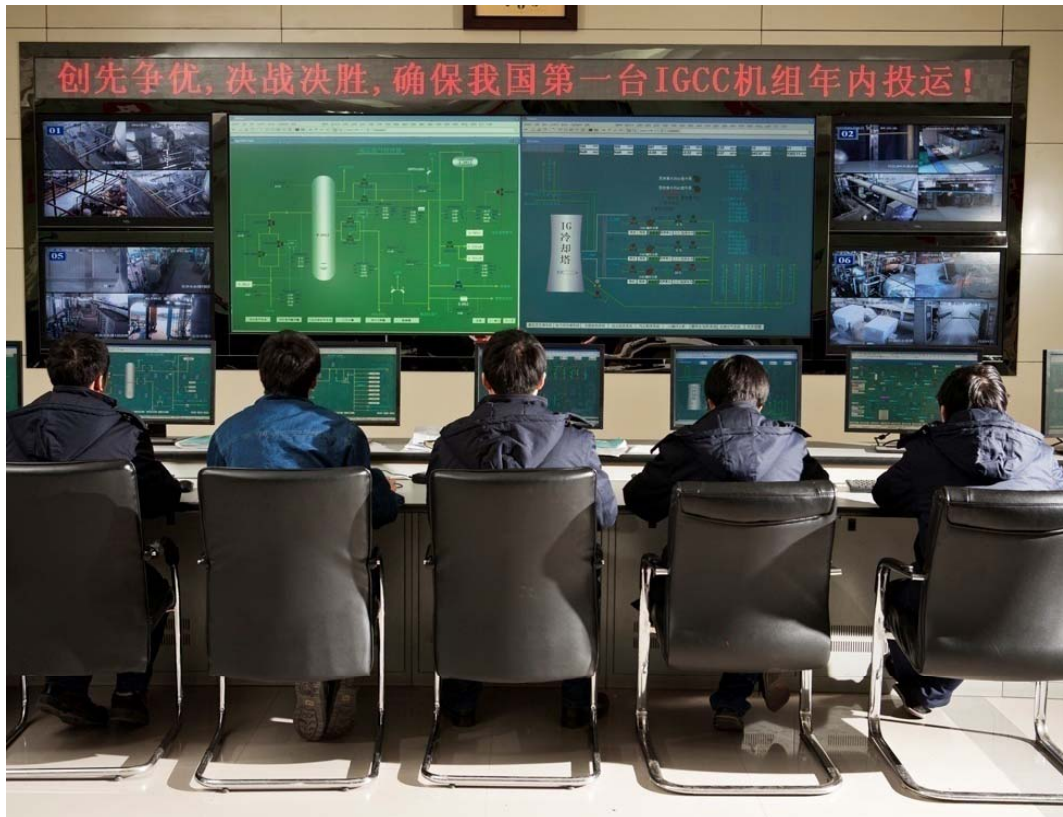
Control Room at GreenGen in Tianjin, China
