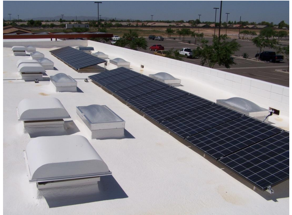
Solar Daylighting with PV
