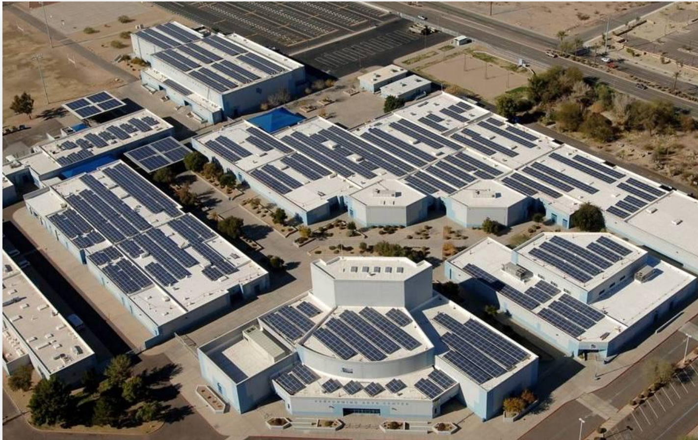
Deer Valley High School, Glendale, AZ - 1 MW installation
