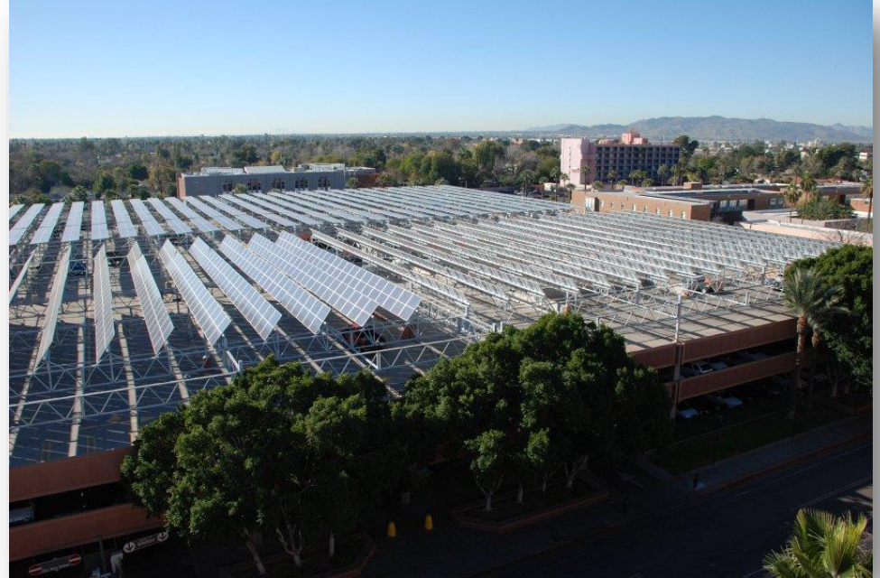
ASU Apache Blvd Parking Structure
