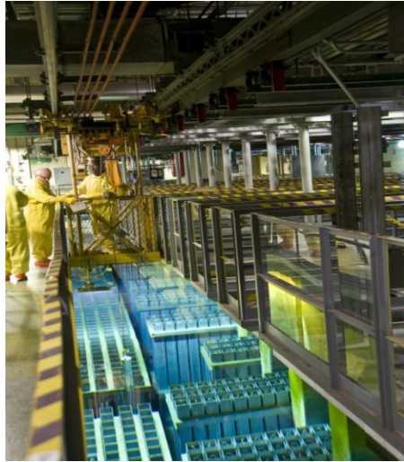
L-Basin SNF Wet Storage Pool
