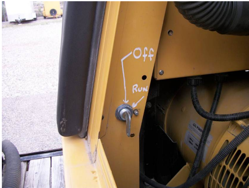
Figure 2. Battery Isolation Switch
