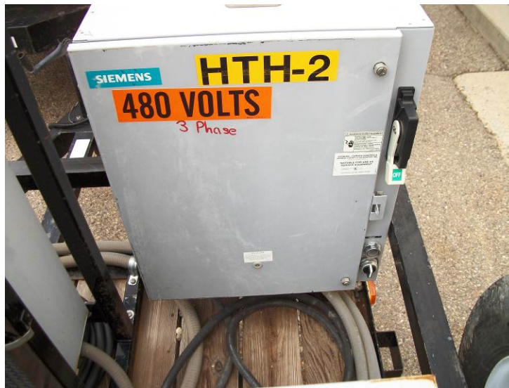
Figure 4. Typical Disconnect Switch
