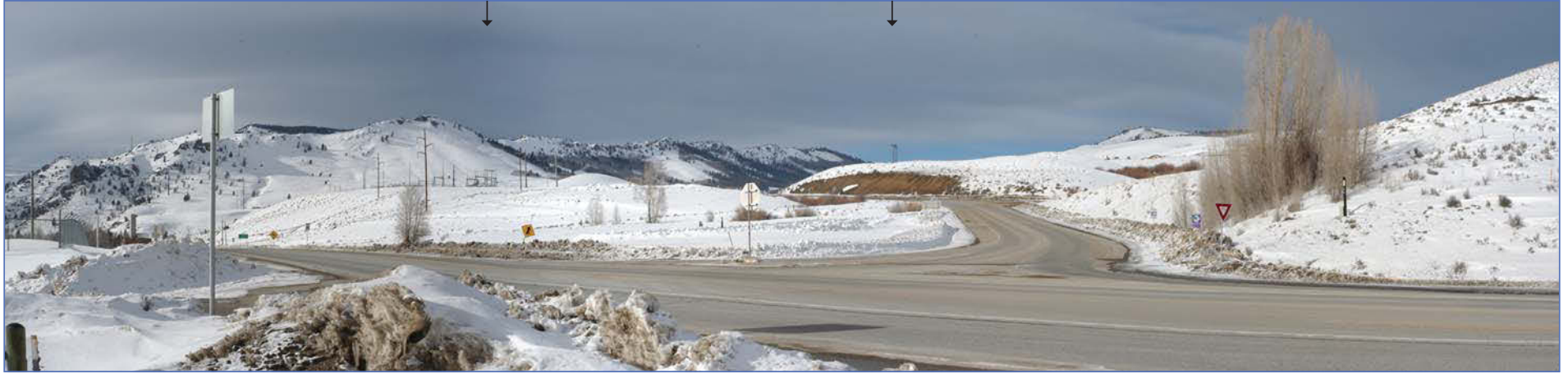
13: Existing Conditions Looking North (March 2009)
