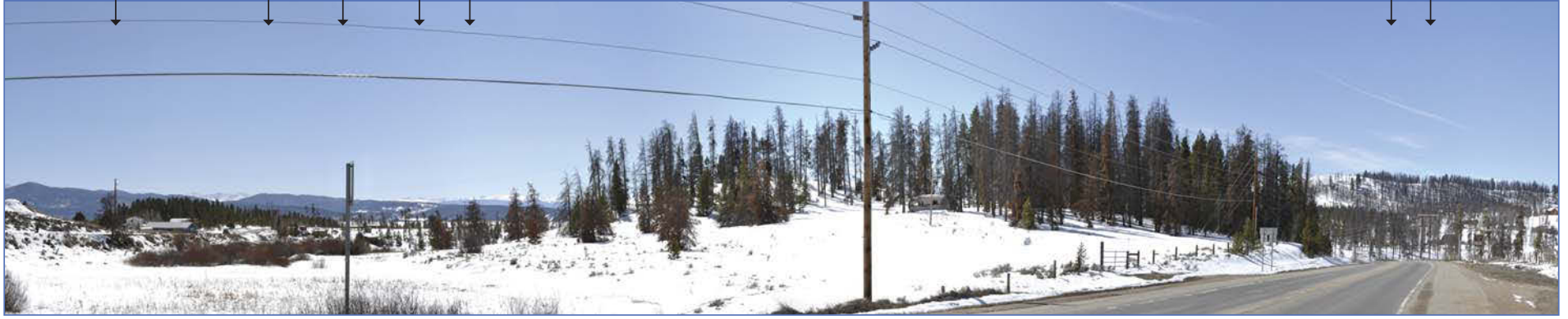
2: Existing Conditions Looking Southwest (March 2009)
