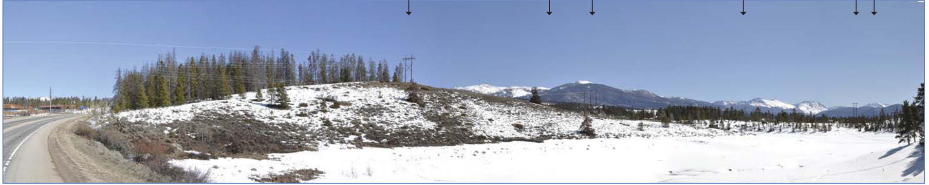
1: Existing Conditions Looking Northeast (March 2009)
