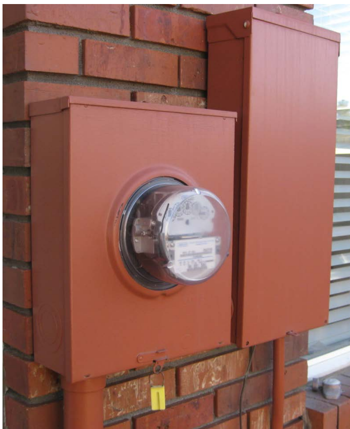
Residential Meter and Disconnect
