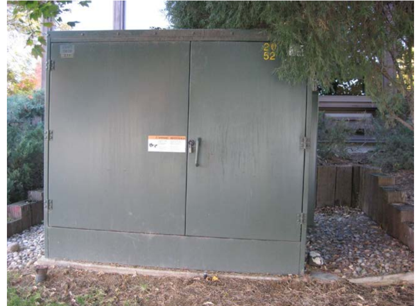
Three-Phase Pad-Mount (13.2 kV to 277/480 V)
