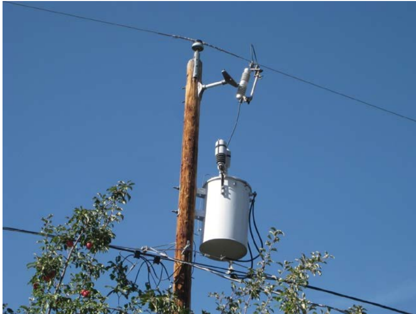
Single-Phase Overhead (7.62 kV to 120/240 V)
