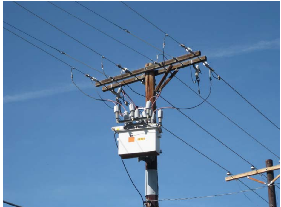
Three-Phase Overhead Recloser
