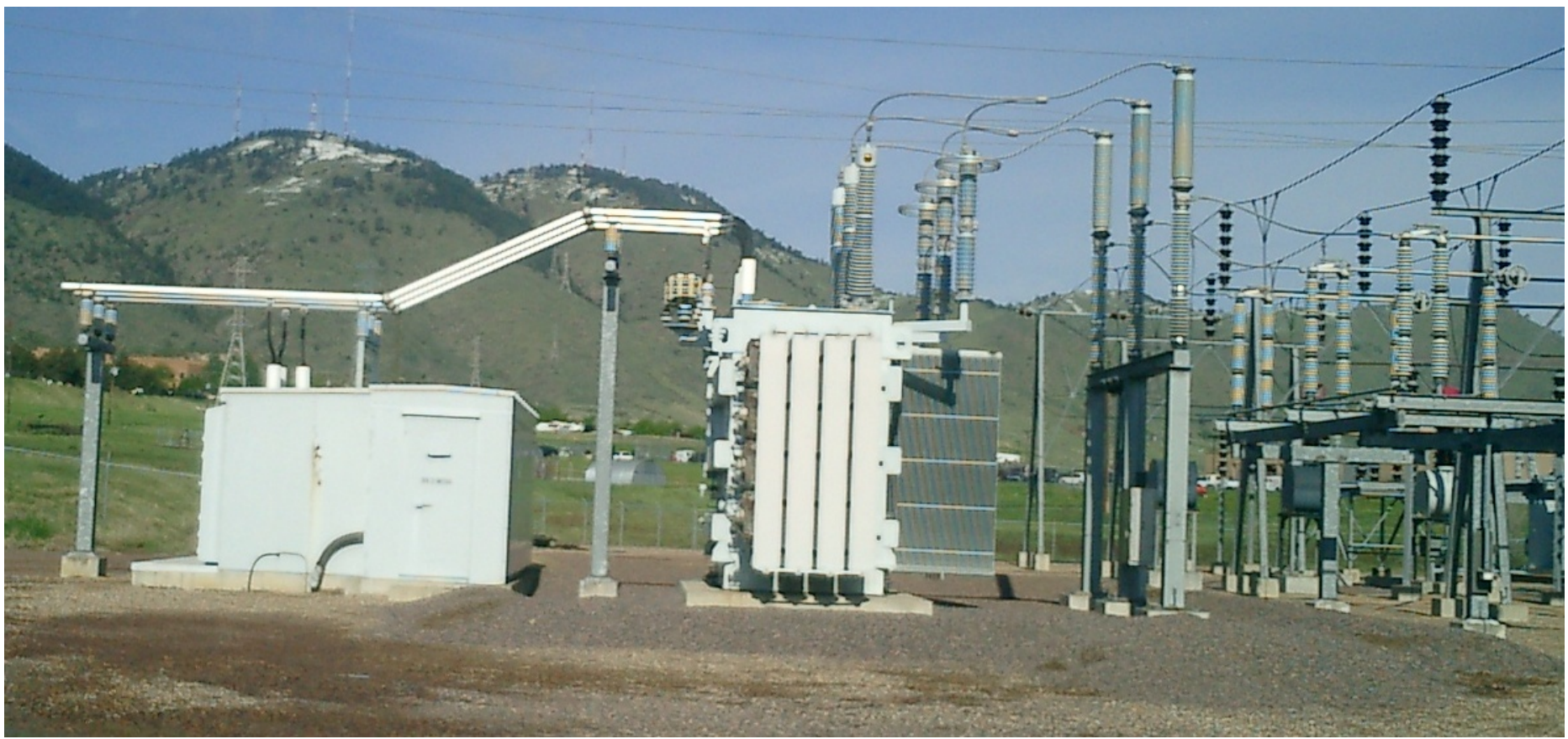
13.2 – 230 kV Transformer
