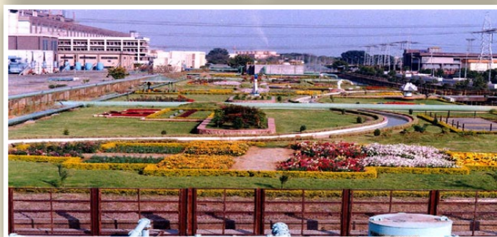
NTPC Korba Power Plant in India
