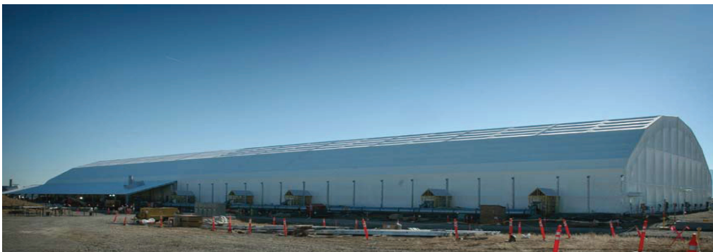
Facility at RWMC
