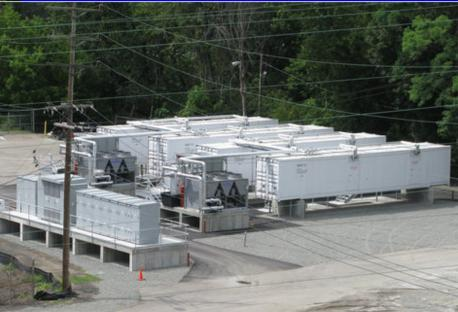
DOE Loan Guarantee – AES / A123: 20MW Lithium Ion Battery for Frequency Regulation in NY-ISO 8MW on Line!
