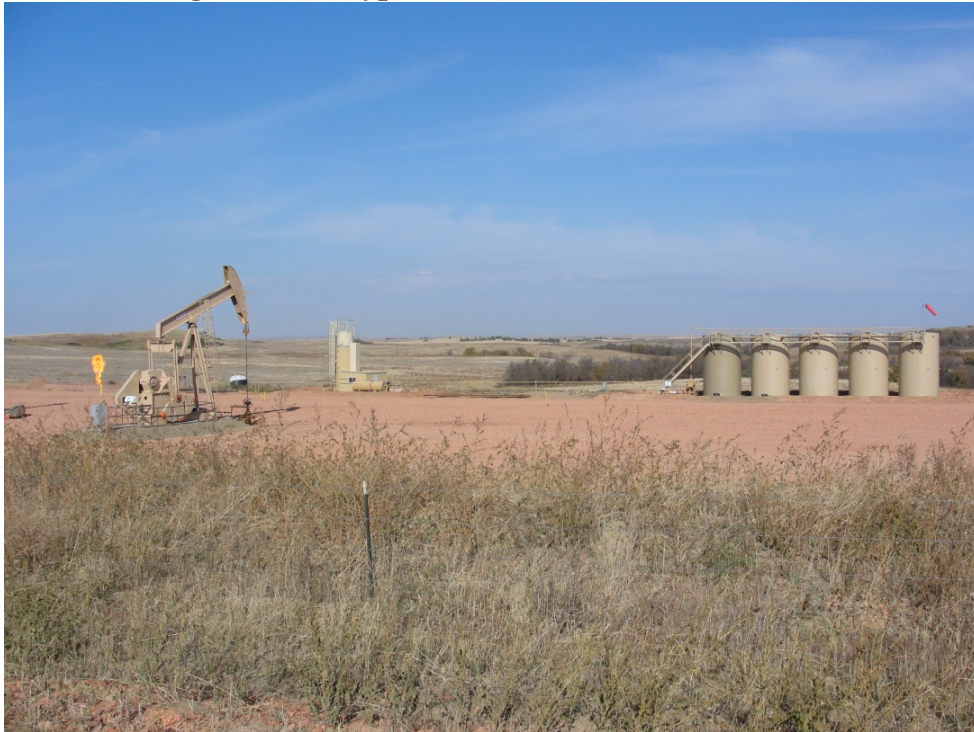
Figure 3-7: Typical Oil Well Pad Site
