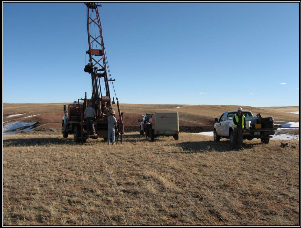
Figure 9. Overview of B9, facing south.
