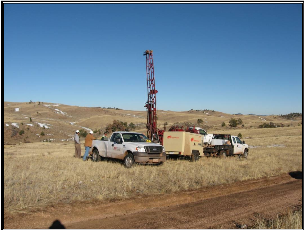
Figure 13. Overview of B13, facing northeast.
