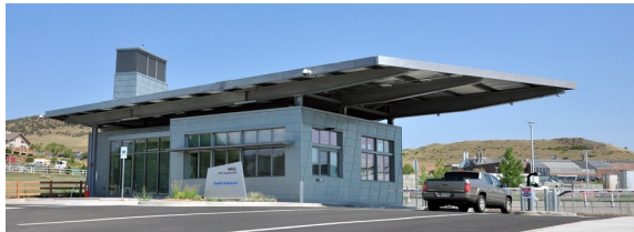
SW, SE and NE exposures
