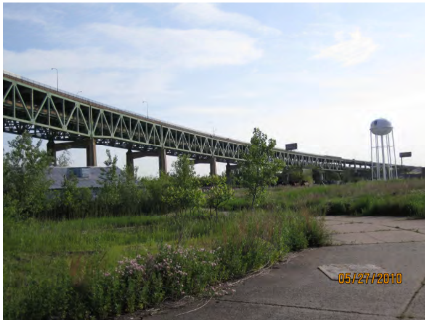
2. Ground View of the Project Site from the Southwest looking to the Northeast
