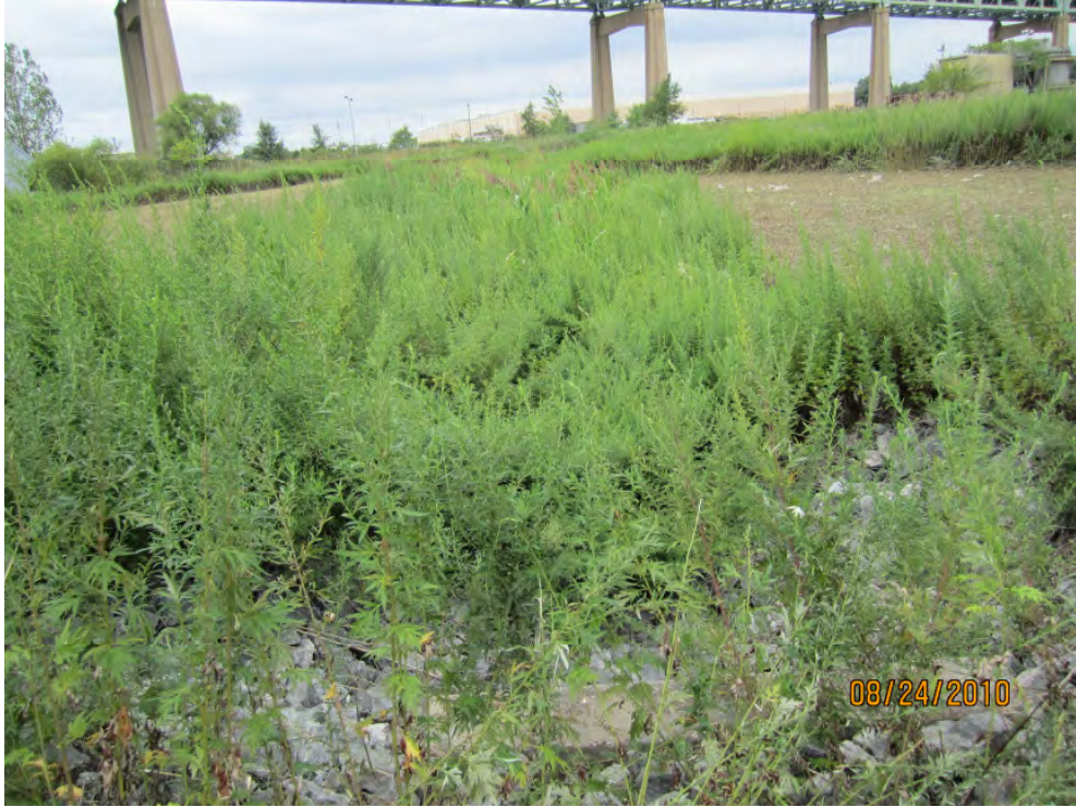
9. Existing inlet at man made swale
