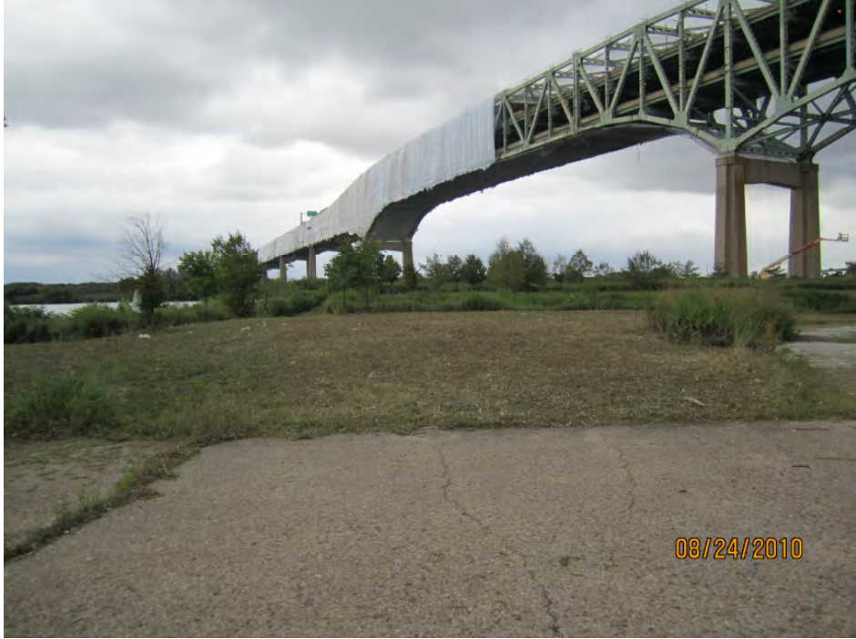
5. Southwestern part of the Project Site
