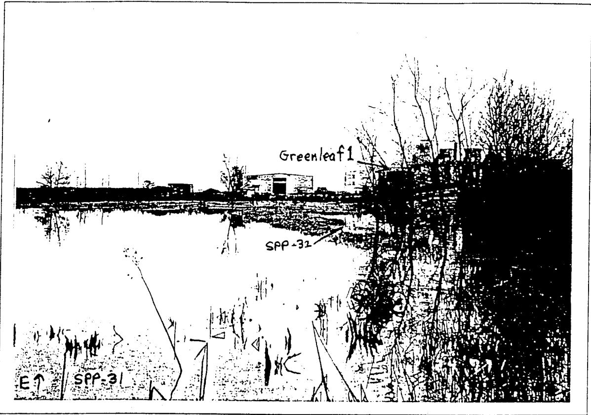
Appendix B-3. Borrow pits (SPP-31 and SPP-32) west of the Greenleaf 1 facility showing ponding during the 1996-97 wet season, January 24, 1997.
