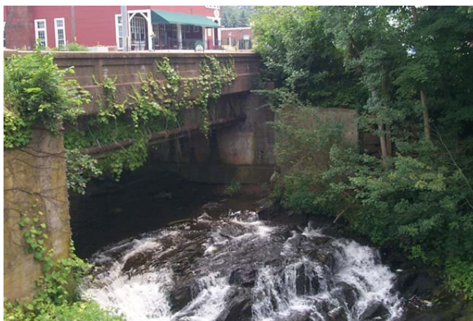
Figure 3.1.15-3 : Photo of Mill Pond Dam Outfall
