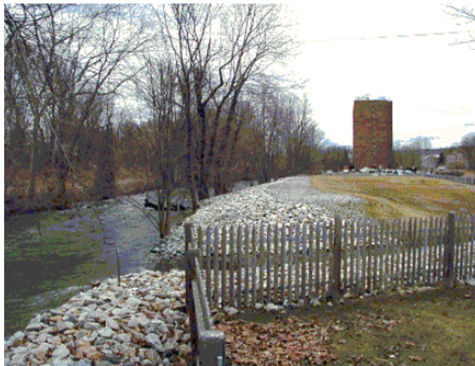
Centredale Manor Restoration Superfund Site
