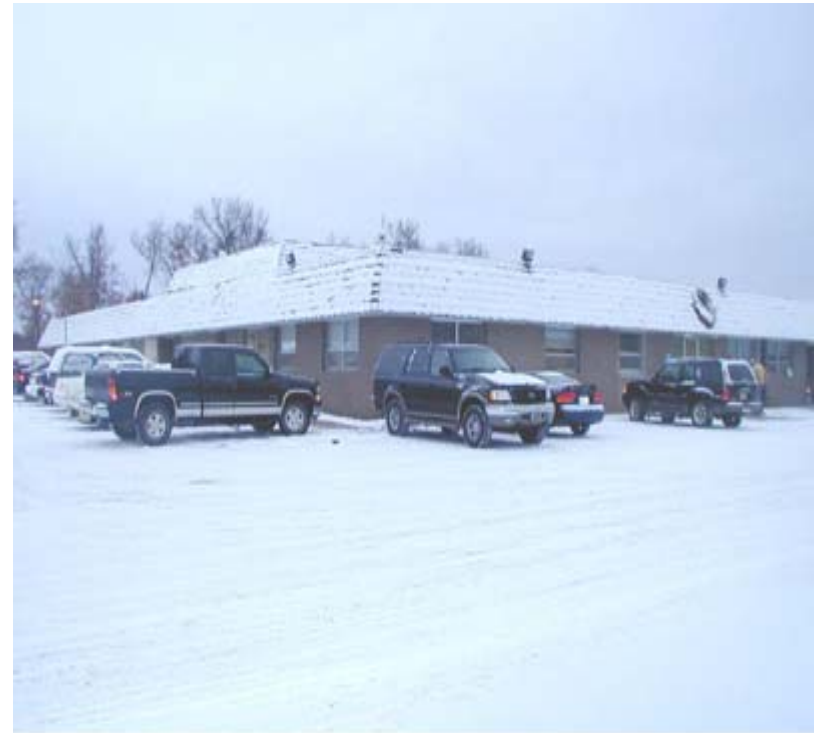
St. Croix Tribal Center
