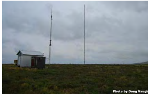
St. George Met Tower (right) and unidentified tower (left)
