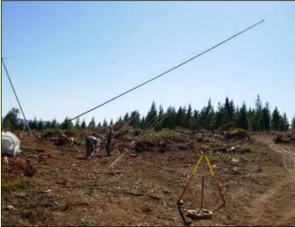
The tower going up.
