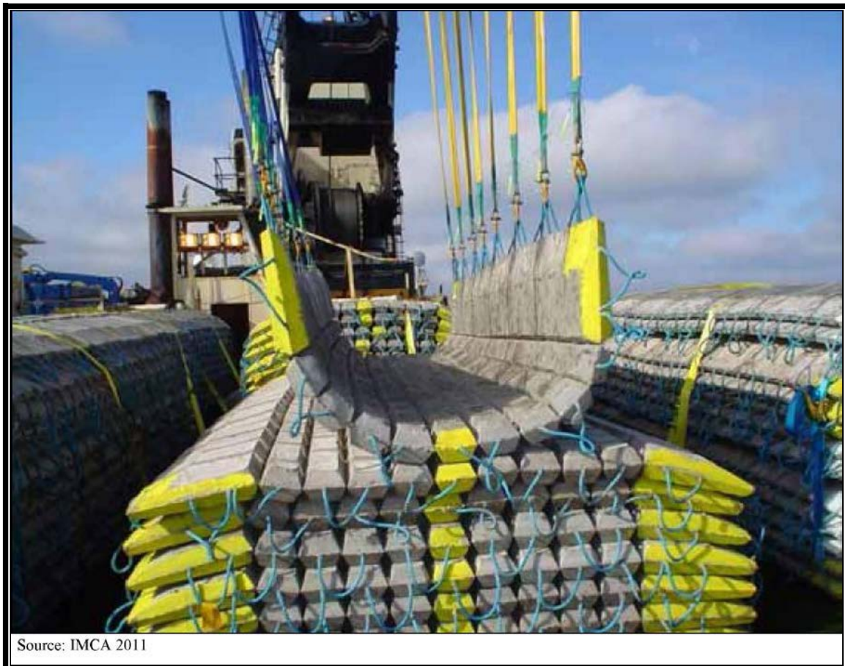
FIGURE 2-4 TYPICAL ARTICULATED CONCRETE MATS
