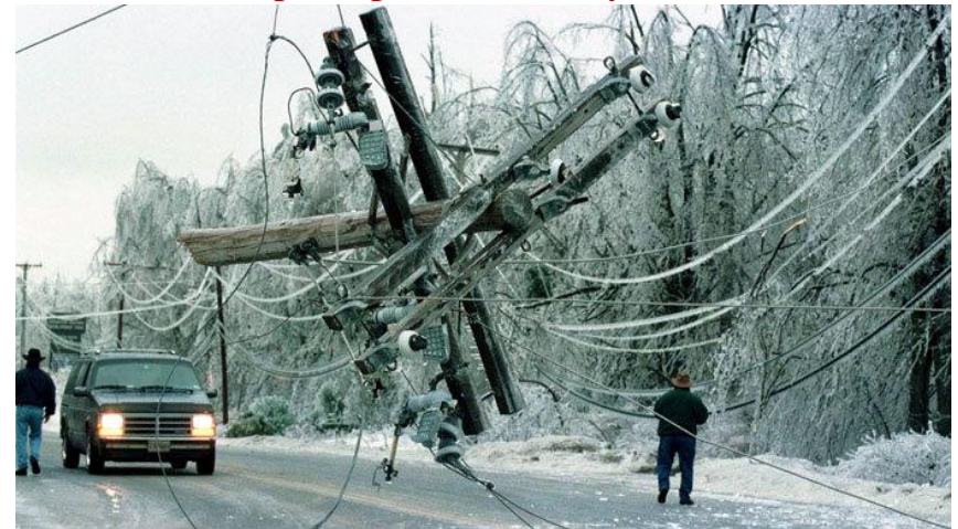
Power poles pulled down by ice storms
