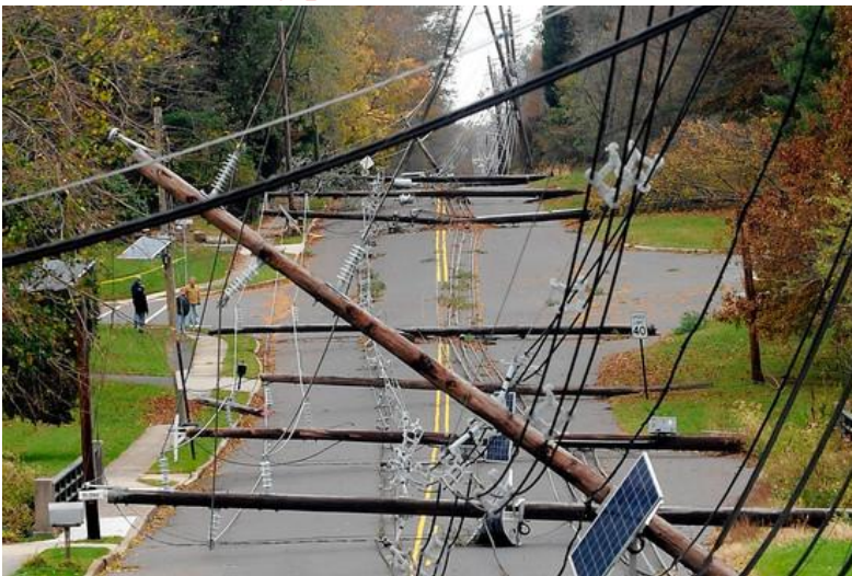
Downed utility poles and wires after hurricane
