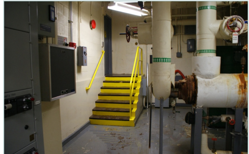
Figure 2-2. MER 7 entrance stairs
