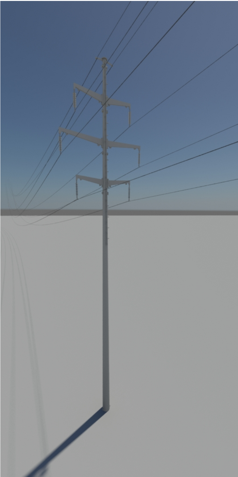
Figure B-3. 3-D Model of Double-circuit Steel Pole Structure Used for Photographic Simulations
