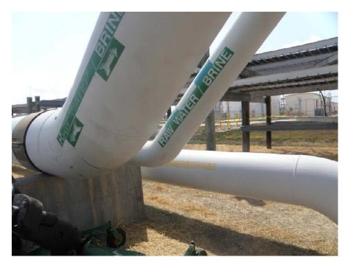
Figure 2-4: Photograph of Section of Pipes Struck by GC1
