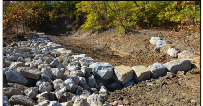
*Construction of a cross-vane is completed while Paddys Run is dry.*
