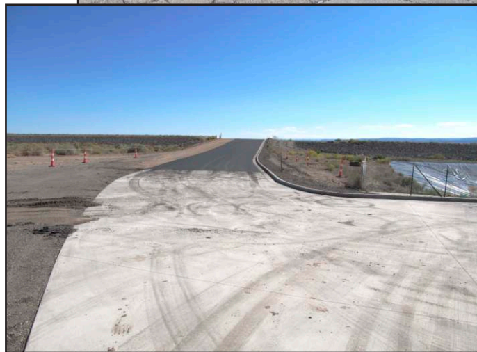
Top: Deteriorated asphalt at the road entering the disposal cell. Bottom: New asphalt pavement at the road entering the disposal cell.
