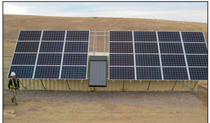
DOE was able to minimize impacts to the habitat of a federally protected mouse and provide the potential for relatively easy relocation by mounting the solar panels on the side of the conex box that houses the batteries and other system equipment.
