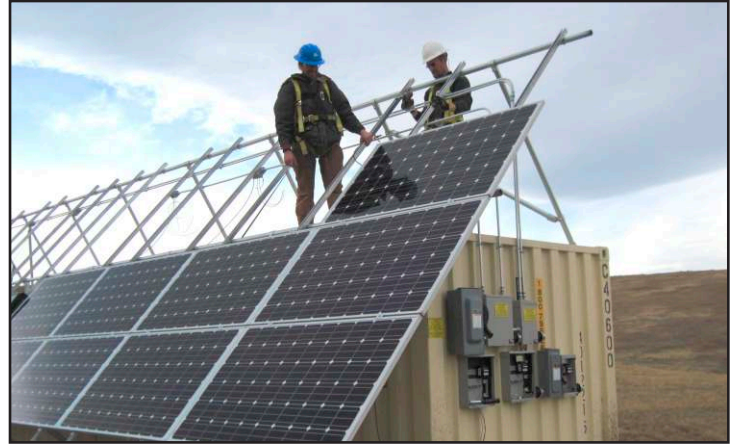
Subcontractor personnel install solar panels and other infrastructure on a 40-foot conex box that houses the batteries and control equipment for the 6 kilowatt photovoltaic system that powers the ETPTS groundwater treatment system.
