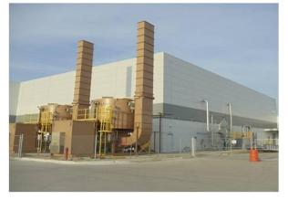
Figure II - 27: The Regenerative Thermal Oxidizer (RTO) by the separator facility.
