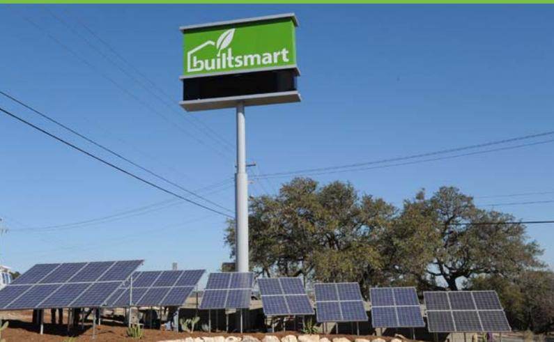
This 11.28-kW PV system was built in 2010 for a net-zero solar model home that was certified as a Level 3 Solar Home by Build San Antonio Green. Photo from Solar San Antonio, NREL/PIX19479
