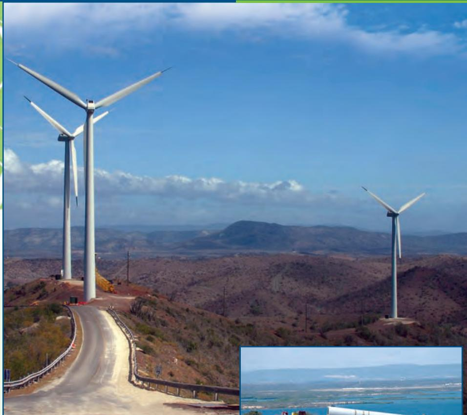
These photographs chronicle the installation of the wind turbines at John Paul Jones Hill, Guantanamo Bay. The four wind turbine towers are about 185 feet high. The blade lengths are 90 feet. The top of the blades are about 275 feet off the ground. The blades rotate at a maximum of 22 RPM, or a rotation every three seconds. This translates to a blade tip speed of 140 mph.
