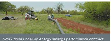
Work done under an energy savings performance contract enables Dyess Air Force Base to use Abilene's effluent water for irrigation, saving 160 million gallons of potable water and \$300,000 a year. Fusion-welded polyethylene piping connects Abilene's effluent supply lineto a holding reservoir on the base.
