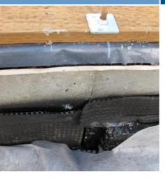
This foundation moisture management approach uses a dimpled-plastic drainage plane and damp proofing on the exterior side of the foundation wall. Landscape filter fabric keeps soil from clogging the gravel around the perforated drainage pipe. A gasket keeps moisture from migrating up through the footing into the treated sill plate.
