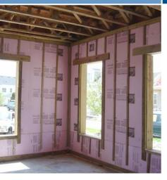
Masonry walls are insulated with interior rigid insulation.
