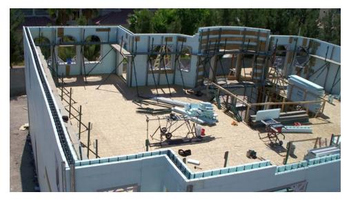
Insulated concrete form (ICF) walls form a solid thermal boundary for the NextGen 2009 home in Las Vegas. (Photo source: iShow.com, Inc.)
