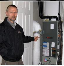
This builder points to a mechanized damper on a fresh air intake to the HVAC air handler. The damper can be set by a timer (shown above) to open allowing fresh air to be pulled into the air handler by the fan, also operated by the timer. This draws fresh air into the house at regular intervals.
