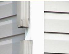
Install flashing at roof valleys and edges and install rain gutters to guide water off roof and away from house. Make sure the downspouts are connected and extend to at least 3 feet from the house. (Photo source: EPA, photo by Terry Brennan)
