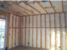
(1) Batt insulation. (2) Blown-in insulation. (3) Foamed-In-Place. (Photo source: Sam Garst) (4) Here, spray foam is applied along the underside of the roof deck to provide a conditioned and non-vented attic space for ducts and air handlers.
