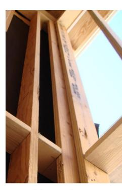
Using dry wall clips or a 1x nailer strip to avoid the third stud in corners provides more room for insulation and reduces lumber.
