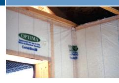
Centex of Northern California used a system it calls "zero defect" wall insulation in homes in San Ramon to help achieve energy savings of almost 40% over the Building America benchmark. It includes 2x6 framing to accommodate R-23 blown fiberglass in walls for more consistent fill than fiberglass batts, R-38 in the ceiling to cover ducts, and careful caulking and sealing of all joints and penetrations to reduce air leakage.
