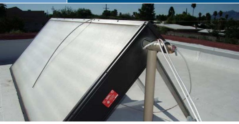
A Sun Earth Copperheart CP 40 integral collector storage solar hot water system is mounted on the roof's flat surface.
