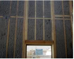
Insulation in non-vented attics is applied directly under roof sheathing. In this example cellulose and carefully sealed joints are used to form a conditioned and non-vented attic. (*Photo source: Pulte Homes*) Note, permeable insulation can only be used at roof decks in unvented attics in the hot-dry/mixed-dry climate zone. In other climate zones, insulation applied along a roof deck in unvented attics must be air impermeable.
