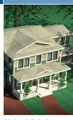
Light-colored roofing, like the roofing specified for the Environments for Living demonstration house at the 2009 International Builder Show in Las Vegas, can help minimize heat gain from solar radiation. Reflective roofs help keep homes (and surrounding neighborhoods) cool and help offset carbon emissions.
