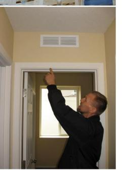
(top) Installing jump ducts from room to room is one way to balance pressures.
