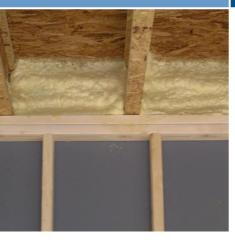
Sealing gaps between floor joists with spray foam provides a good air seal that prevents the flow of heat, cold, and pollutants from unconditioned space to conditioned space.
