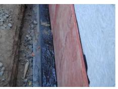
Here, a damp proof coating and exterior rigid fiberglass insulation are applied to the foundation wall below grade
