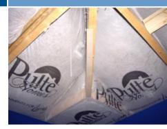
Pulte's unique method of applying attic insulation keeps the blown cellulose right up against the roof line. This insulated attic provides conditioned space at the air handler and ducts at around 80°F instead of the 150°F temperatures found in uninsulated Las Vegas attics.
