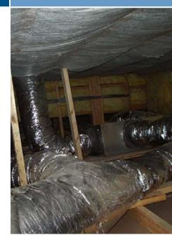
Ducts are located in conditioned space and mastic sealed to minimize heating and cooling losses.
