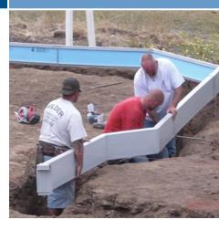
Davis Energy Group of the CARB Building America team developed a new method for insulating slab perimeters that is ideal for extremely hot climates and mixed dry climates. The method, which is still being tested, uses termiticide-treated rigid foam insulation encased in PVC as the form for the concrete foundation.
