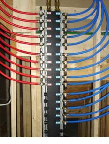
A centrally located manifold water distribution system saves energy by reducing hot water usage.
