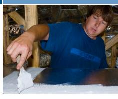
Mastic provides the most reliable duct sealing method. Ducts should be located in conditioned space. (Photo source: BAIHP)
