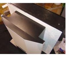
This exhaust fan and electronic controls are designed to ventilate—and could be used to create a slightly negative pressure in—the garage. Ventilation carries pollutants to the outside; negative pressure helps to stop garage air from migrating into attached houses.
