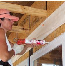
(top) Holes for wiring are sealed with foam.
