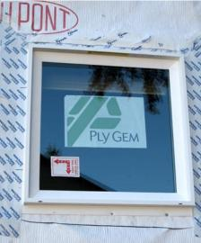
(top) Windows should be flashed in accordance with ASTM E2112-07.
