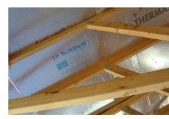
Radiant barriers can significantly reduce solar heat gain through the roof.
