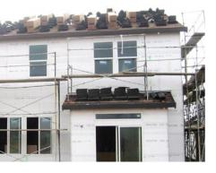
Taped rigid foam insulation can serve as a drainage plane and air barrier as well as a thermal boundary behind a stucco cladding. If using housewrap instead, never apply stucco directly to plastic housewrap. Provide a drainage space to prevent wetting of the housewap or use two layers of textured building paper.
