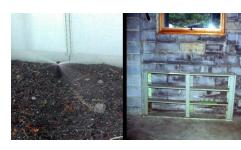
This sprinkler was placed too close to the house's foundation wall. Moisture seeped through the concrete block causing water stains and mold inside. (Photo source: EPA; photo by Terry Brennan)
