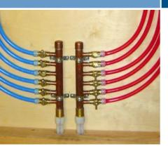
In an NAHB Research Center study, the central manifold hot water distribution system provided hot water to the fixtures more quickly than traditional trunk and branch and remote manifold distribution methods.
