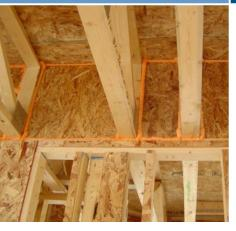
In this figure, OSB and foam form the air barriers to isolate the garage from living space.
