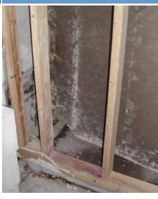
When moisture is trapped inside walls, mold can grow unchecked causing damage to the walls and health impacts for the occupants. (Photo source: EPA; photo by Terry Brennan)
