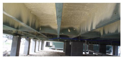
High-density closed-cell spray foam was sprayed between the 2x10 floor joists, in the 2x6 stud wall cavities, and along the underside of the roof decking to air seal and insulate. It also glues the components together to help the homes better withstand hurricane-force winds. All lumber is borate pressure-treated to resist rot and wall cavities are treated with an in-wall pest defense product.
