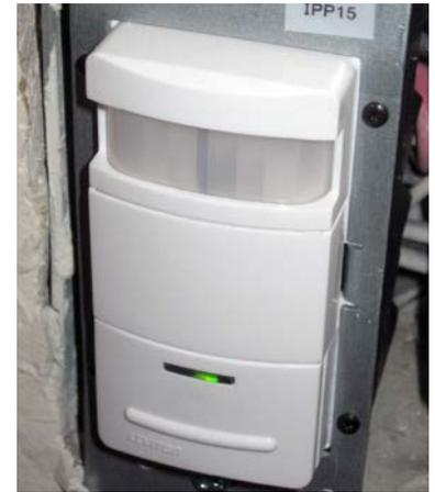
Aerosolized duct sealing (left) helped reduce duct leakage to outside by up to 62%. Lighting controls, like this occupancy sensor (above), helped to automate control and reduce energy consumption.
