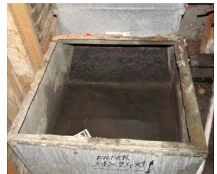
Air sealing at the Sasha Bruce group home in Washington, DC (top), required accessing some tight spaces. The existing plenum (bottom) had 4 in. of standing water from an improperly plumbed condensate line! Replacing and replumbing saved energy and improved indoor air quality.
