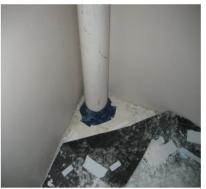
The vertical ventilation pipe runs from the foundation to the roof and serves as a passive sub-slab depressurization system that effectively reduces radon levels in the home. Follow these general steps to construct a passive radon ventilation system.
